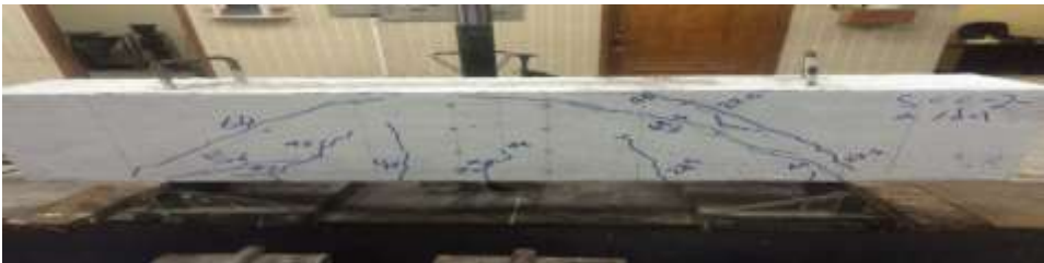
Fig. (5): Crack Pattern for Beam A-1
