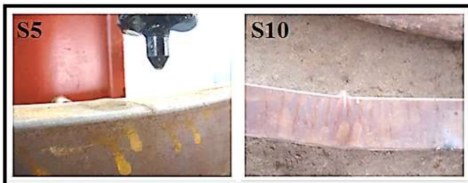
Fig.(8) Failure patterns for columns S 5 and S 10
